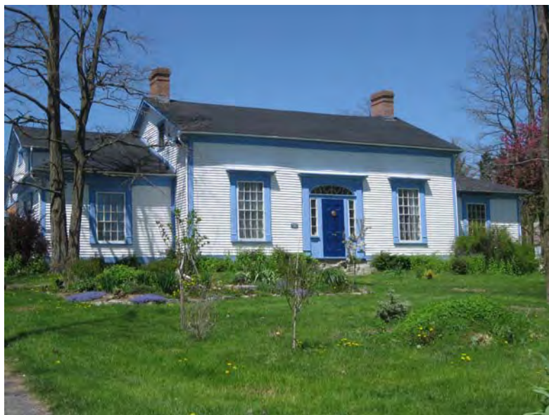
The Peter Davy House (370 Academy Street, c.1811-1819) displays a Neo-Classical interpretation of the Ontario Cottage style through its attention to refined detailing, such as on the window and door surrounds.
