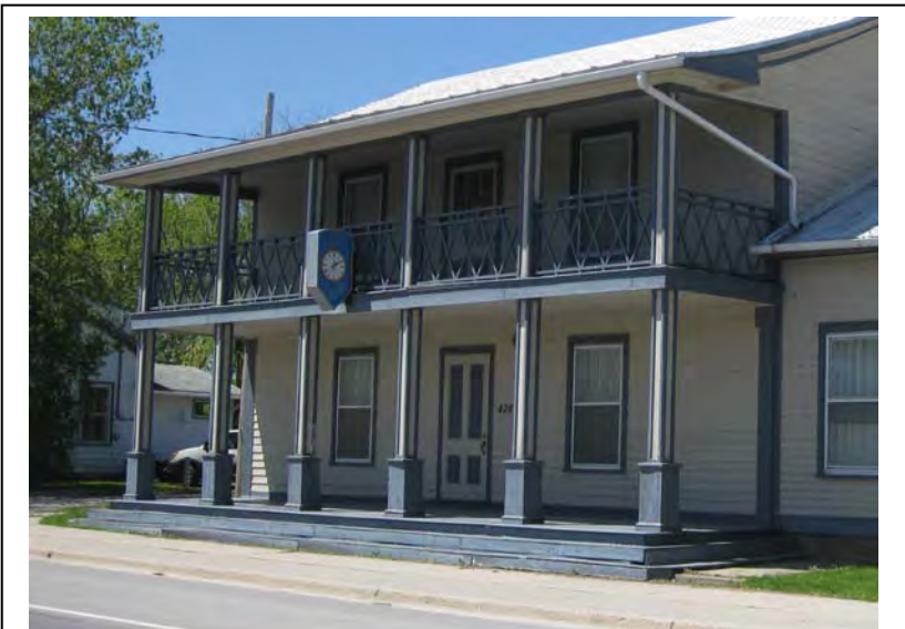
The double verandah of the E.D. Priest Store (428 Main Street) is characteristic of commercial structures in the Village of Bath. The verandah extends the length of the main façade and features suitable wooden detailing, typical of the commercial Regency style.
