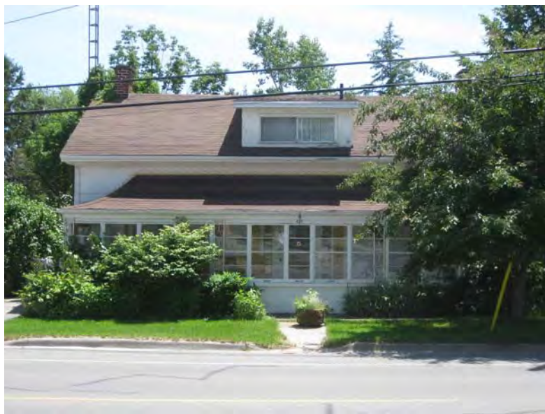
The Dr Roderick Kennedy House (429 Main Street, 1855) is a vernacular interpretation of the Regency Cottage style. Of particular interest is the bell cast verandah roof with detailing and cladding finished to appear like ashlar cut stone. The shed dormer and enclosure of the verandah were later interventions.
