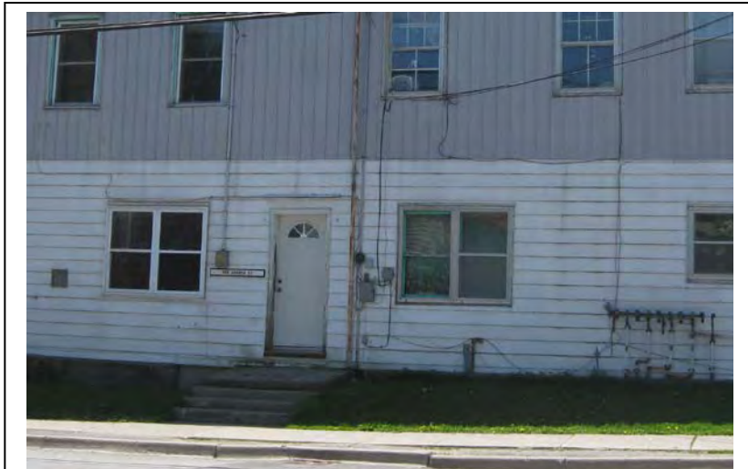
The placement of utility meters on the Church Street façade of 195 Church Street negatively detracts from its cultural heritage value. The utility meters clutter building, interrupting the symmetry of the façade. The rear of the building would be a more appropriate location for utility meters.
