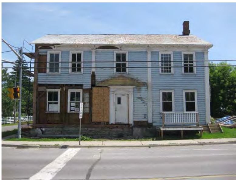
The Ham House (353 Main Street, c.1819), seen in a state of restoration (May 2012), is one of the best examples of the Neo-Classical style in Upper Canada. It was included in John Blumenson's Ontario Architecture (1989). Significant details include the pilasters and palmette molding in the entablature.
