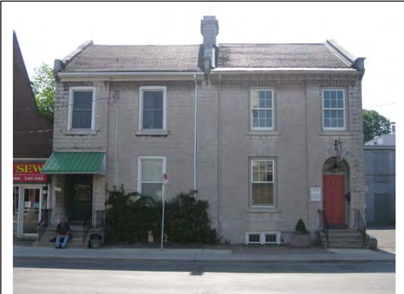
Heritage-quality windows are integral to the cultural heritage value of many heritage resources. On the right, heritage-quality windows have been conserved. On the left, windows have been replaced, with a significant impact on the physical or design values of the heritage resource.
