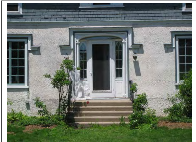
The main entry door of the Reeves Brothers House (452 Main Street) has been identified as a heritage attribute because of its physical or design value.
