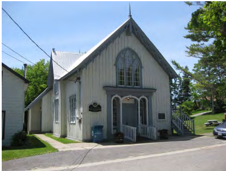
The Layer Cake Hall (193 Davy Street, 1859) is a unique Carpenter Gothic style structure including bargeboard, triple-arch entry, and board and batten cladding.
