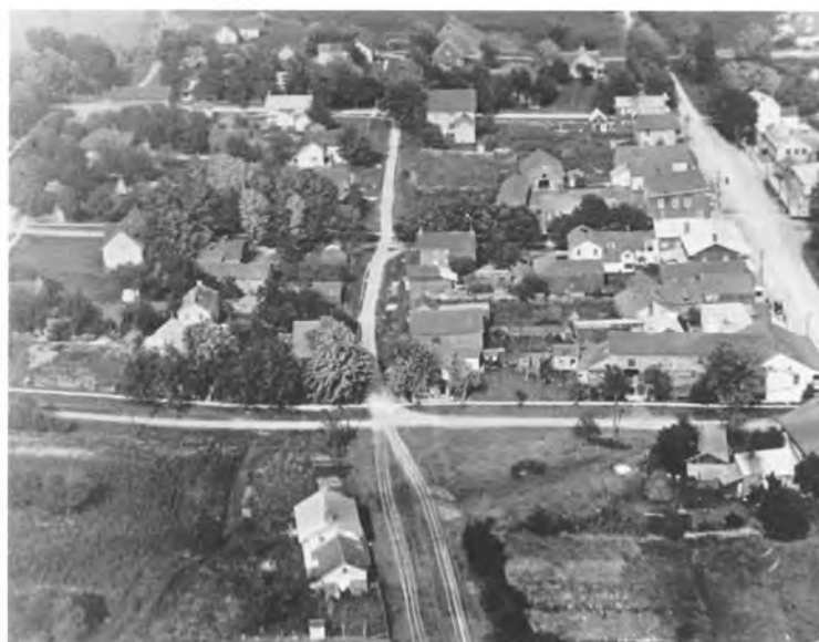
AN AEROPLANE VIEW OF BATH, ONT. COPYRIGHT, CANADA, 1920, BY MC CARTHY AERO SERVICE LIMITED, TORONTO
