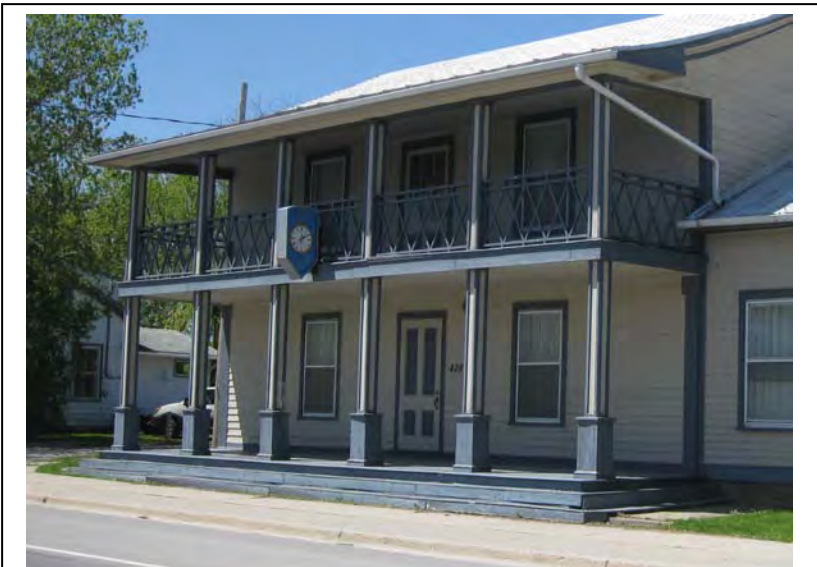
The double verandah of the E.D. Priest Store (428 Main Street) is characteristic of commercial structures in the Village of Bath. The verandah extends the length of the main façade and features suitable wooden detailing, typical of the commercial Regency style.
