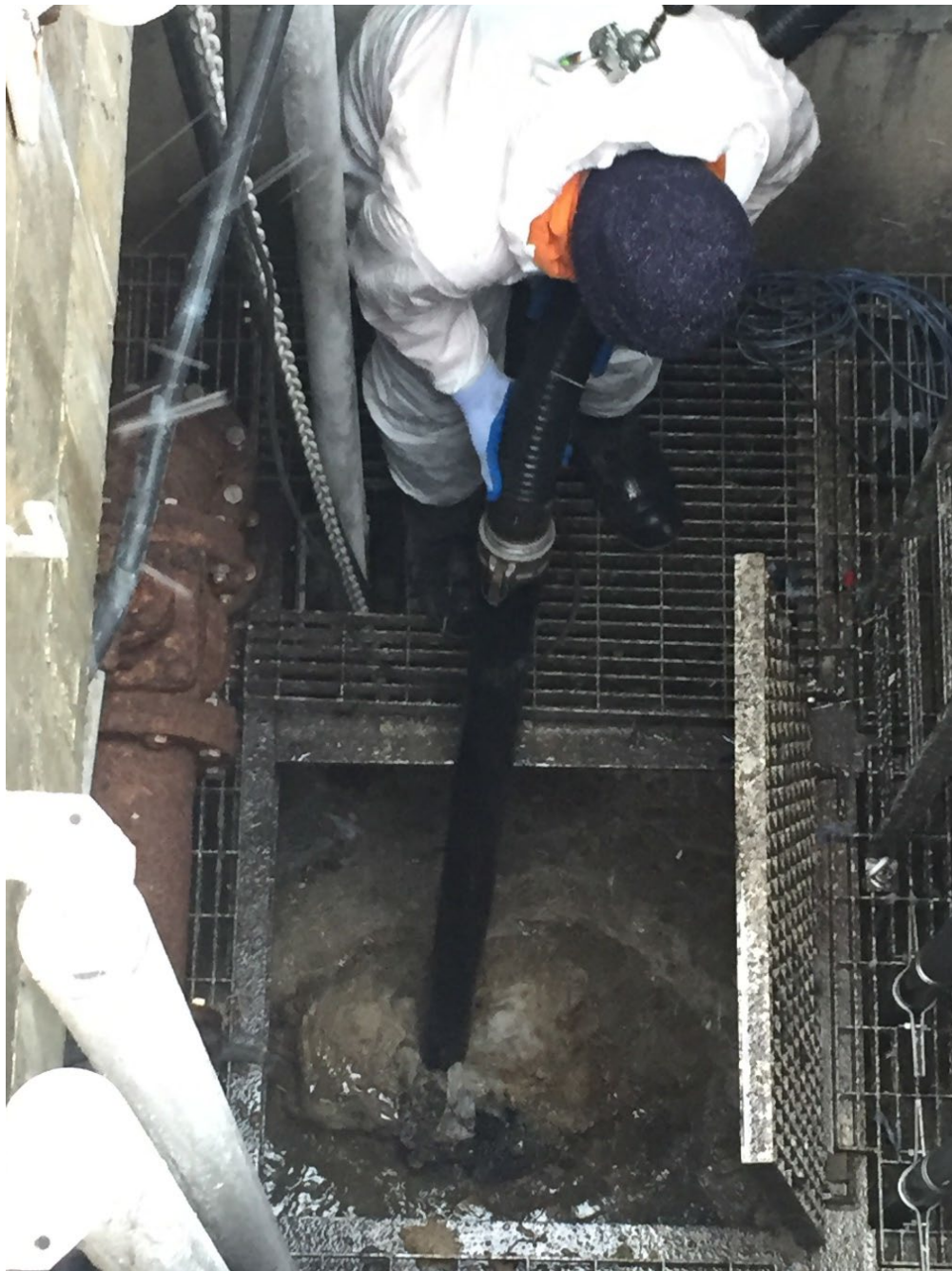
Figure 3 Cleaning of Islandview SPS
