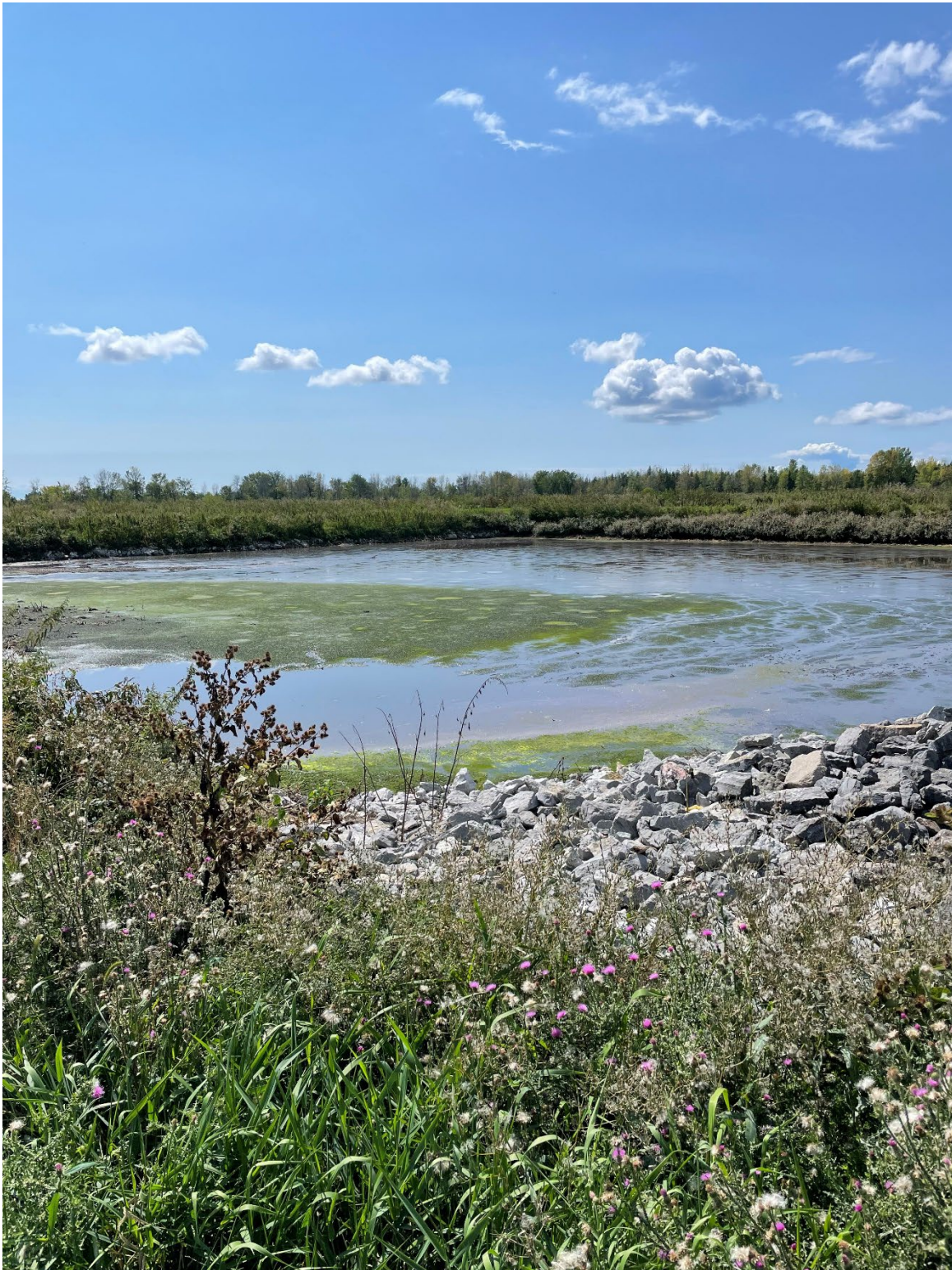
Figure 7 AWPCP - Solids lagoon
